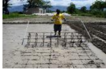
Roller markers are most efficient to mark a grid in only one passage
